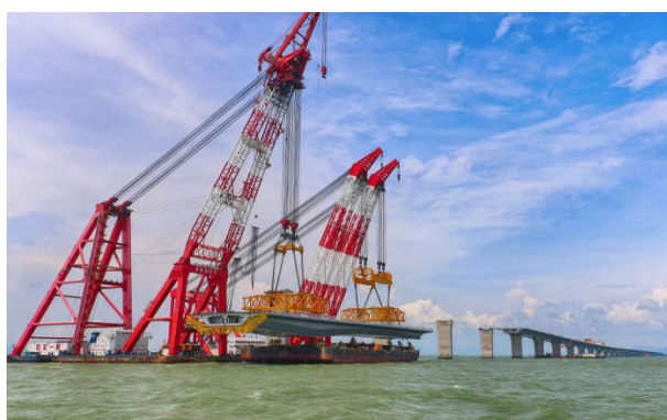
Figure 3. Erection of a full span steel box girder
