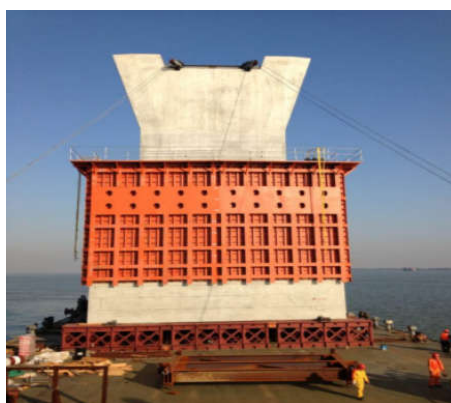
Figure 8. Steel cofferdam for connection between pile cap and pile
