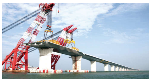
Figure 13. 4000t Floating crane for erecting girders
