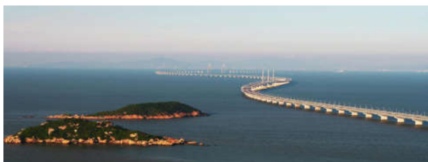
Figure 1. Layout of the completed Hong Kong-Zhuhai-Macao Bridge
