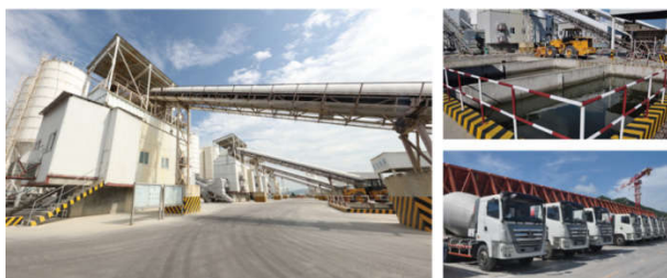
Figure 11. Concrete batching plant
