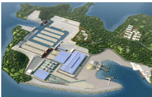
Figure 6. Layout of fabrication factory for tunnel elements
