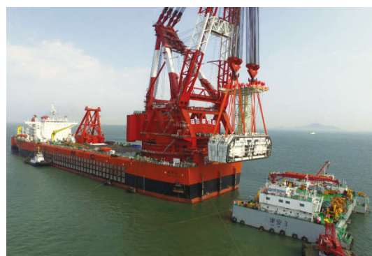
Figure 14. 12000t Floating crane for installing tunnel closure element
