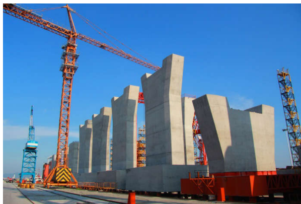
Figure 2. Precast pile-cap and pier units
