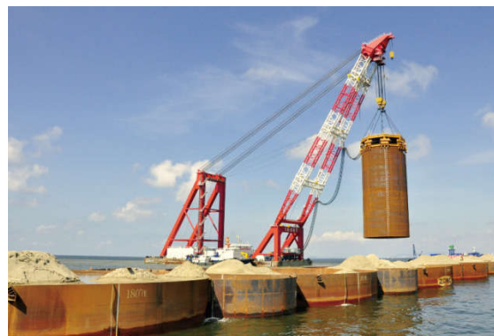
Figure 5. Steel cylinder for drilling into the ground to form island
