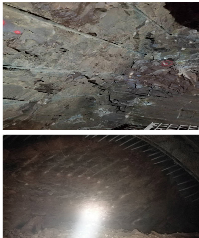
Figure 2. Renderings of Yanshan tunnel exit after blasting
