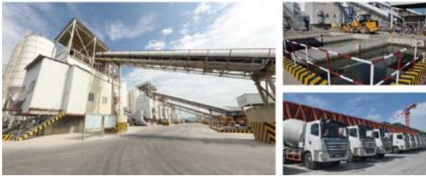
Figure 11. Concrete batching plant
