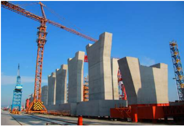
Figure 2. Precast pile-cap and pier units
