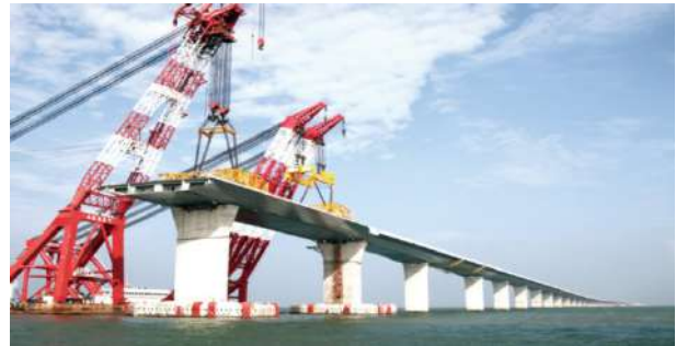
Figure 13. 4000t Floating crane for erecting girders
