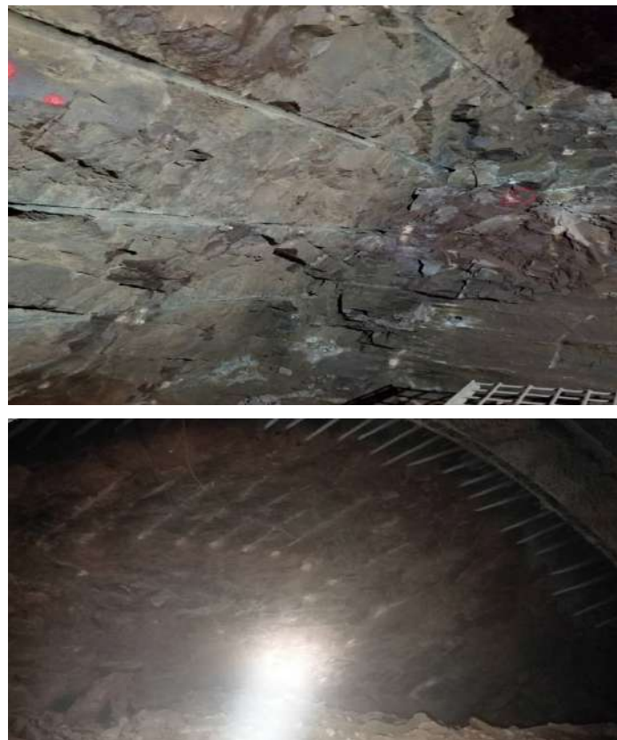
Figure 2. Renderings of Yanshan tunnel exit after blasting
