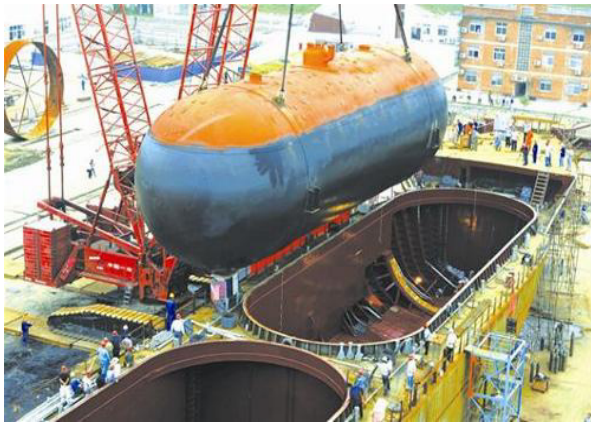
(b) The deck tank
