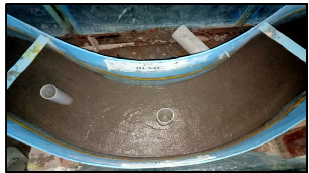
Figure 5. Showing the pier positions for 4 th Run in Bend – 2
