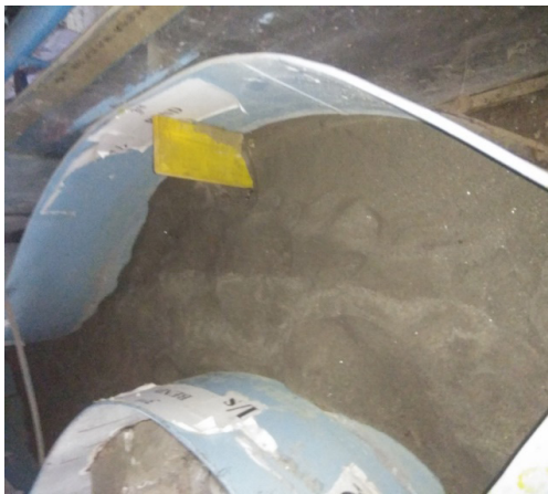
Figure 3. Installation of spur dyke
