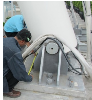
Figure 15. A survey revealing that the existing bases of the legs have no major deficiencies in alignment and leveling following the EQ indicates that the foundation system likely held its integrity.
