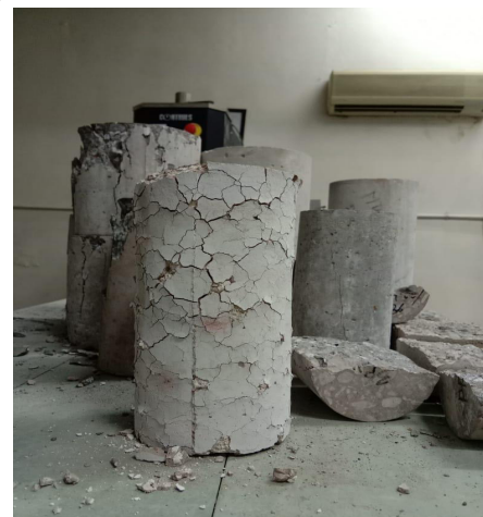
(b) Cylinder with control mix with severe spalling
