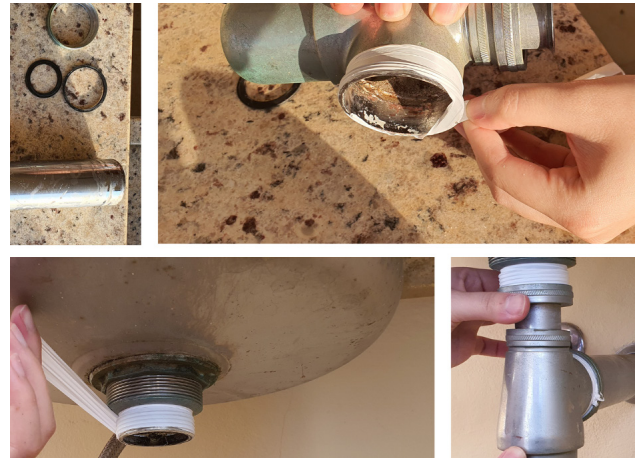
Figure 1. Sink trap maintenance process
