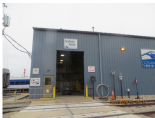
Figure 5. The NCDOT Capital Yard Maintenance Warehouse
