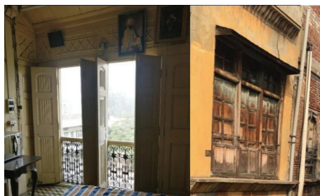
Figure 7. Typical windows in Katras
