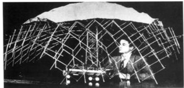
Figure 6. Pantograph for the folding itinerant theatre. Pérez Piñero, 1961
