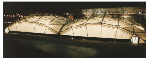
Figure 13. Swimming pool roof in San Pablo sports area in Seville, Escrig, Sánchez and Valcárcel
