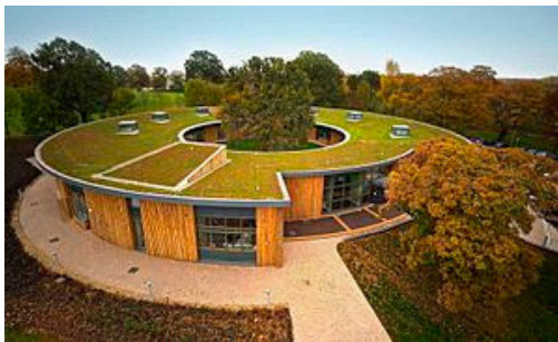
(a) Extensive green roof
