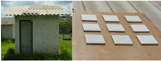
Figure 1. Low sloped roof with exposed specimens and detail of investigated samples
