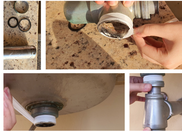
Figure 1. Sink trap maintenance process
