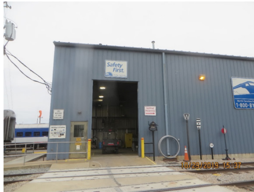
a) Exterior of Warehouse
