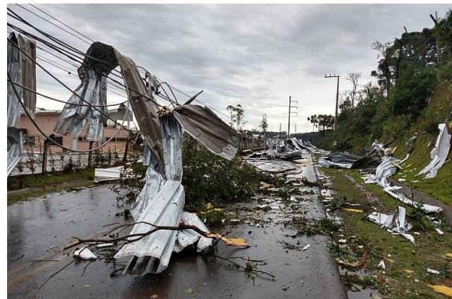
Figure 2. Santa Catarina State was the most affected by the cyclone; On image, area registration destroyed in Chapecó [1] . Photo: Chapecó City Hall (SC)
