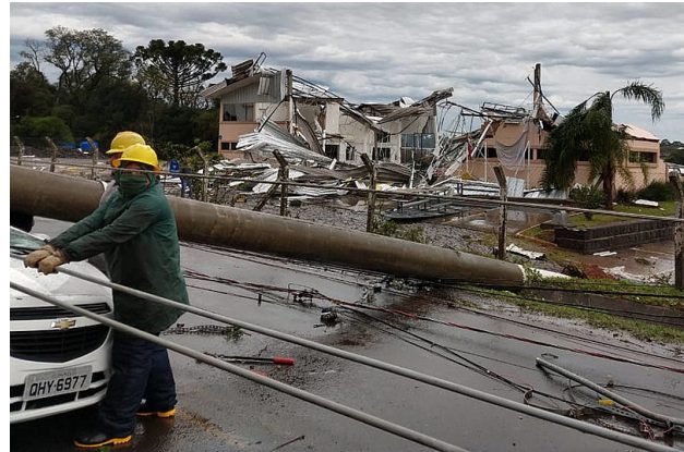
Figure 1. Picture of the destruction caused by the cyclone pump in an urban area of the county of Chapecó in Santa Catarina, which is one of the hardest hit [1] . Photo: Chapecó City Hall (SC)
