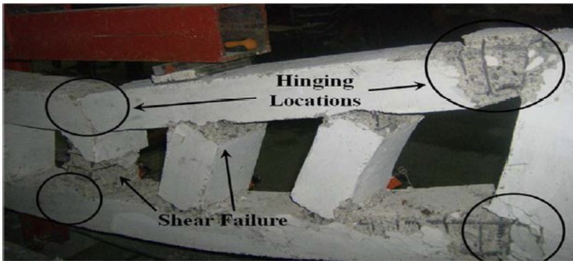
Figure 18. Failure between openings in reinforced concrete beams.
