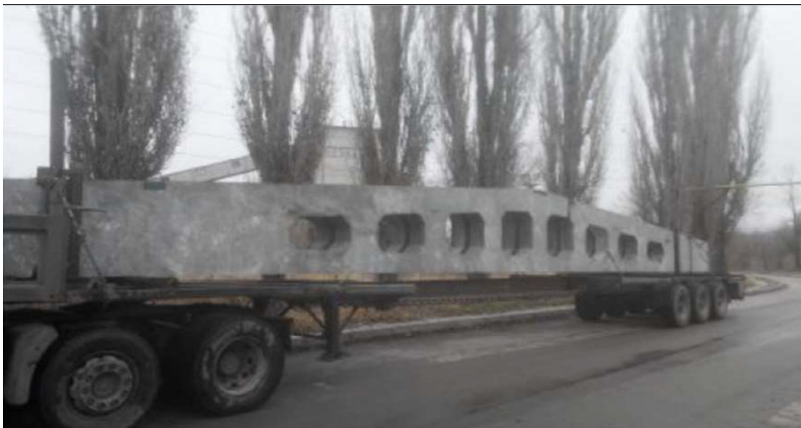
Figure 1. Reinforced concrete gable beam with multiple openings [5] .
