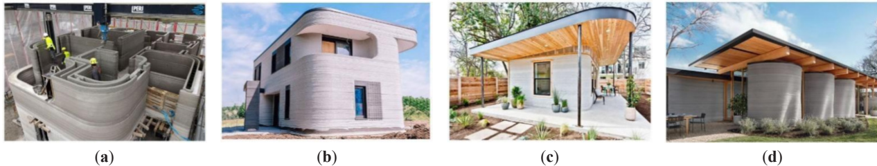
Figure 1. Examples of 3D printed houses. (a, b) The first 3D printed concrete house in Germany [15] ; (c) 3D-printing of affordable concrete houses in Mexico [16] ; (d) 3D printed concrete house in Texas [17] . All houses are characterised by the production of vertical walls using 3D-printing; slabs and roof are made with conventional formwork or other materials.
