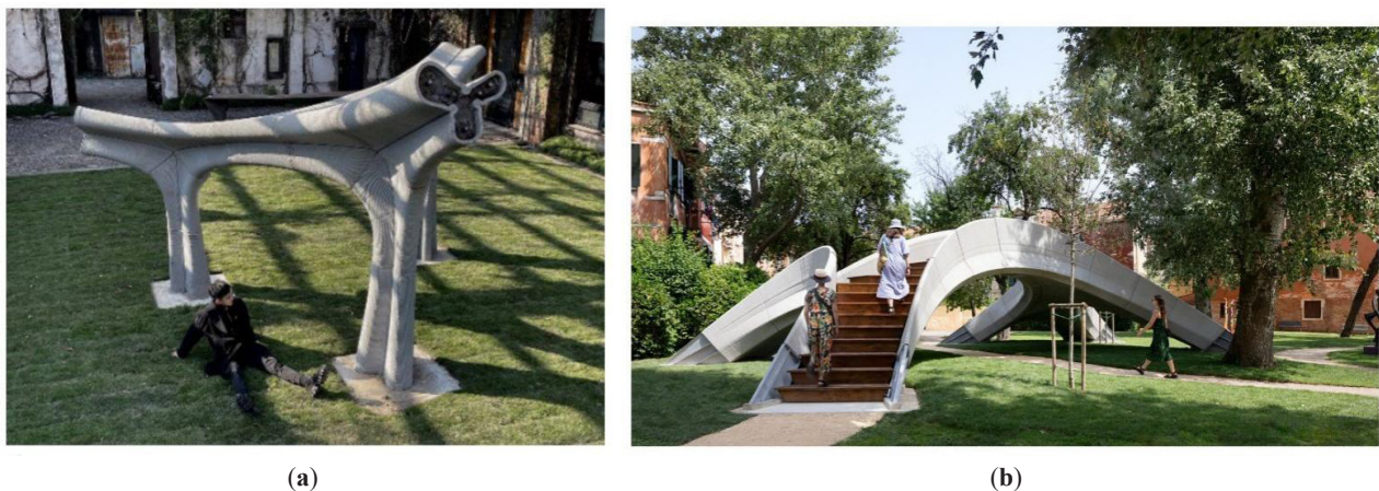
Figure 2. (a) An example of a 3D printed pavilion, showing the use of 3D printed concrete to produce a complex structural geometry [14] ; (b) 3D printed concrete bridge, where the geometry is adapted in such a way that the bridge is entirely in compression [13] .
