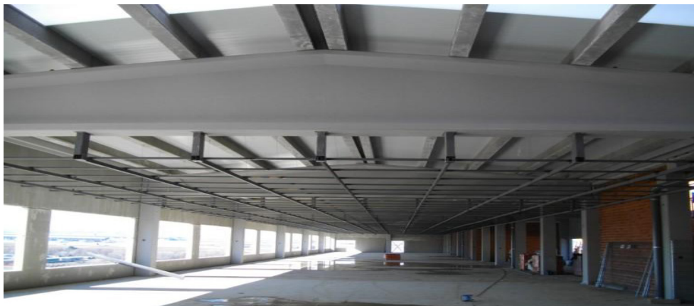
Figure 1. Reinforced concrete gable beams [1] .
