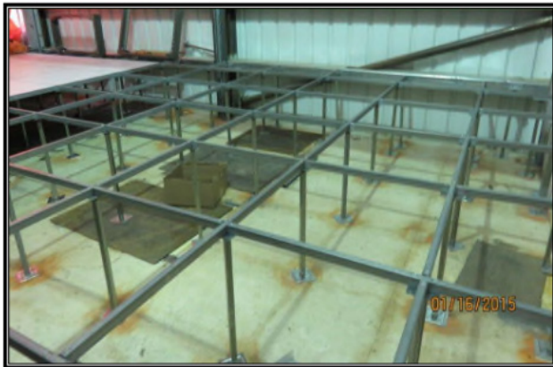
Figure 4. Raised Floor Framing Layout
