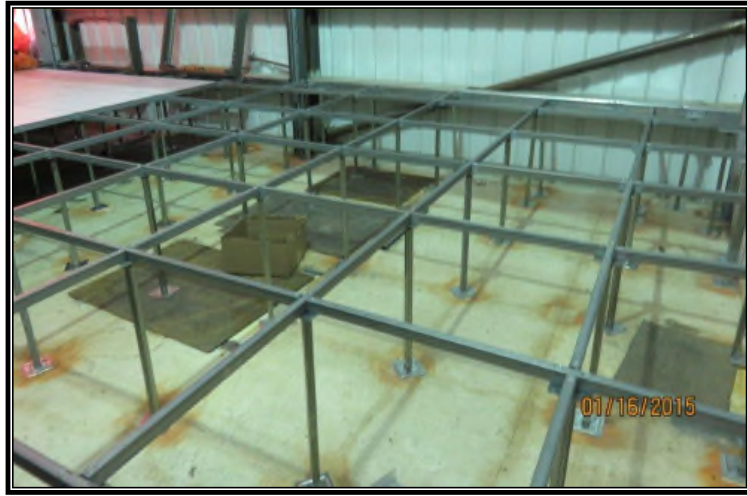
FIG (4) RAISED FLOOR FRAMING LAYOUT
