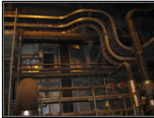
b) Suspended Electrical Cable Trays
