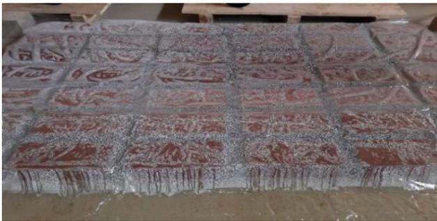
Figure 3. Curing with plastic sheet
