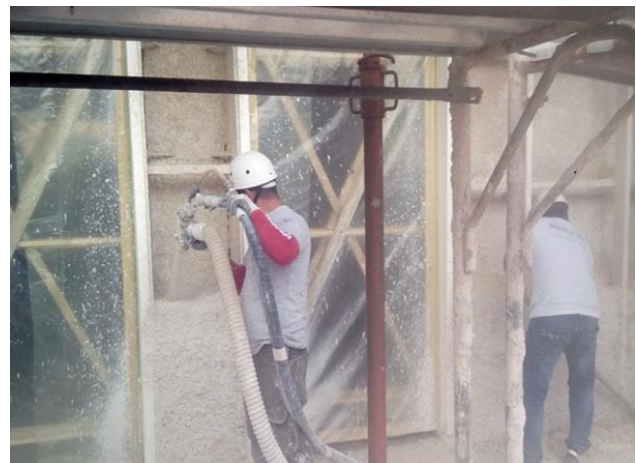
Figure 4. Hemp lime concrete sprayed application
