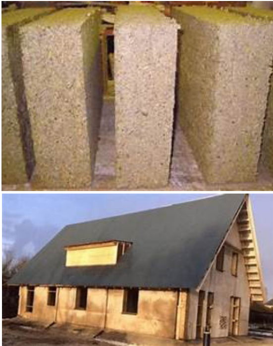
Figure 7. Construction with Hempcrete
