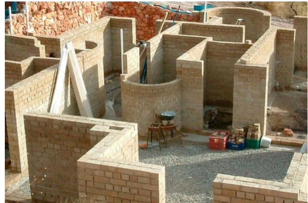
Figure 3. Walls with hemp clay bricks
