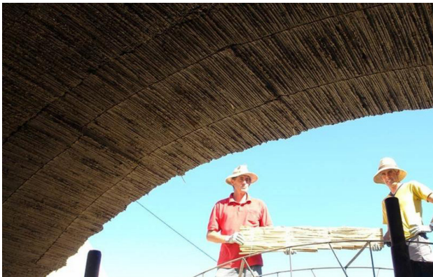
Figure 5. Structural vault of hemp concrete
