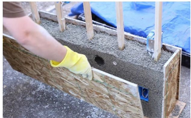
Figure 8. Form packing of hempcrete
