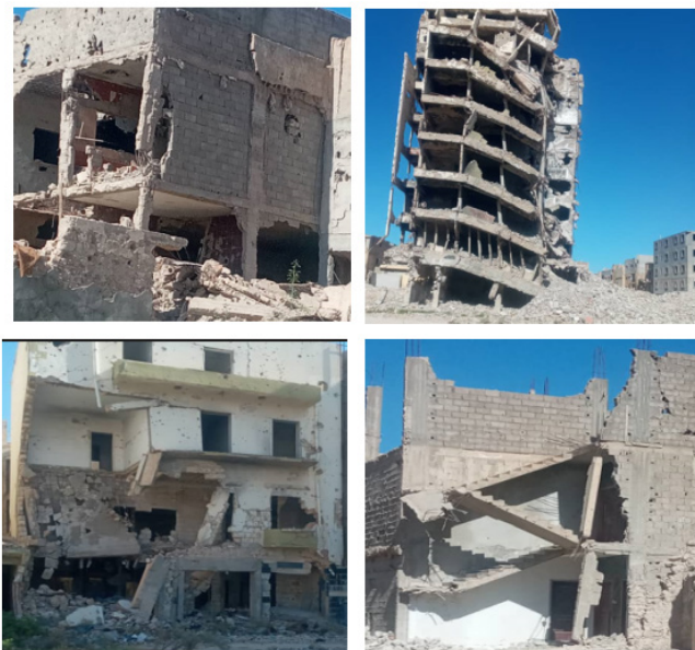
Figure 5. Examples illustrating buildings of completely demolished or severely damaged.
