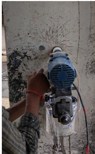
(e) Concrete core cutting
