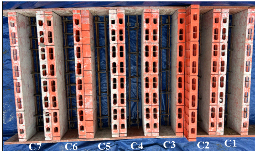
Figure 3. The formwork and reinforcement for the columns have been created.
