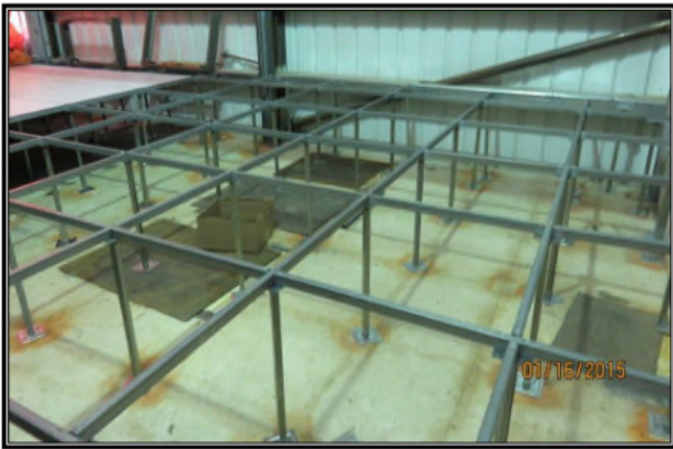
Figure 4. Raised Floor Framing Layout
