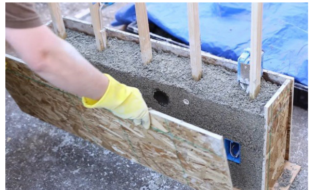
Figure 8. Form packing of hempcrete
