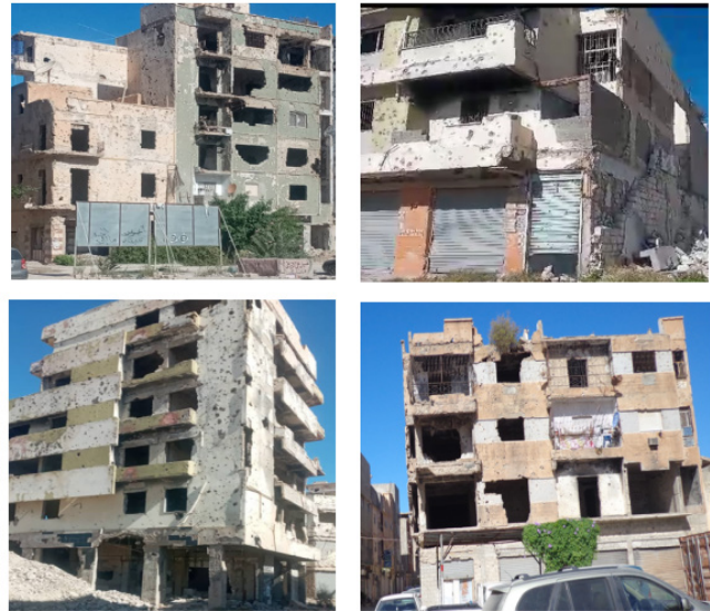
Figure 3. Examples illustrating buildings with medium damage.
