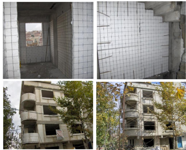
Figure 10. Use 3D panels as infill walls with good connections with the peripheral frames.
