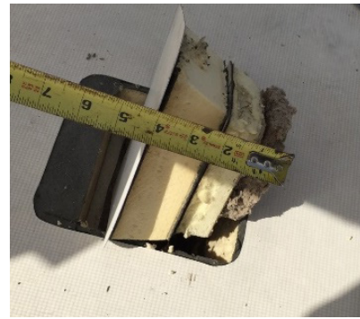
Figure 4. Roof "A" North Side
