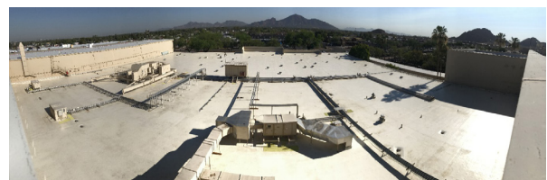
Figure 9. Roof “A” After
