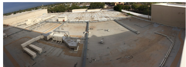
Figure 8. Roof “A” Before
