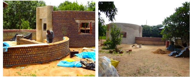
Figure 2. The first two-bedroom bungalow made of entirely sand filled plastic bottles
