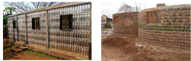
Figure 3. Different bottle walls built in developing countries with various bottle configurations
