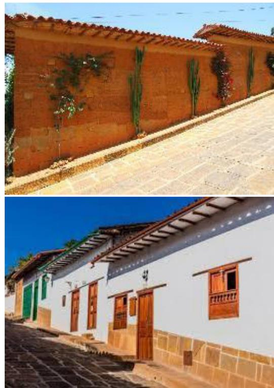
**Figure 2.** City of Barichara in Colombia. Constructions with rammed earth walls [6].
