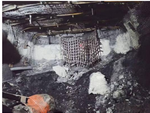
Figure 12. Field photo of the haulage gateway at 159 m ahead of M16.
