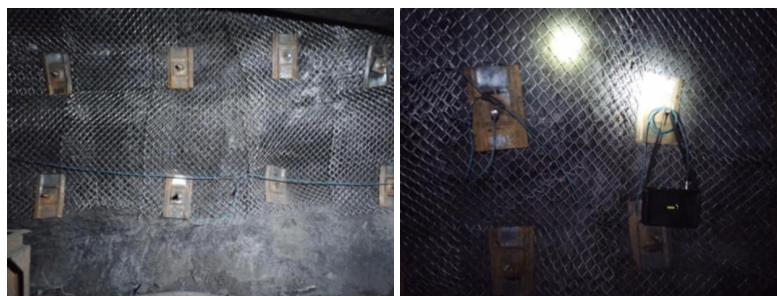
Figure 13. Vibration sensor layout plan and photos.
