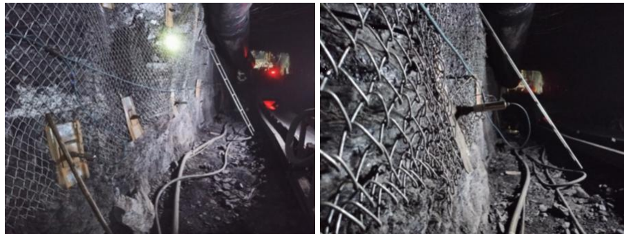
Figure 10. On-site vibration sensor layout and installation photos.
