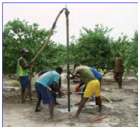
Figure 8. Mud drilling [9] .
