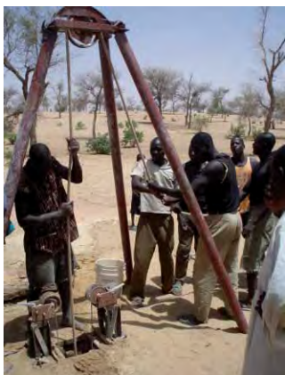
Figure 6. Percussion drilling [9] .
