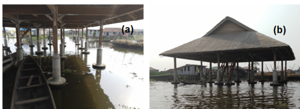
Figure 27. (a) Reinforced concrete piles installed in place of wooden ones. (b) View of the constructed lake habitat model.
