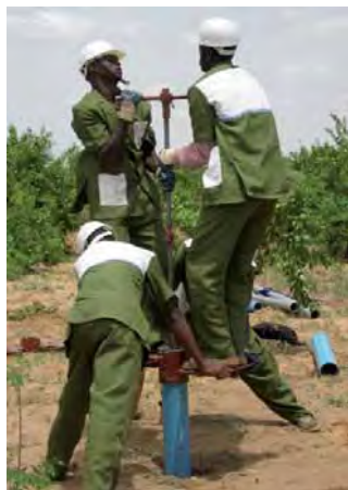
Figure 5. Auger drilling [9] .
