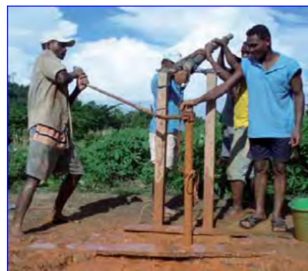
Figure 7. Percussion drilling [9] .
