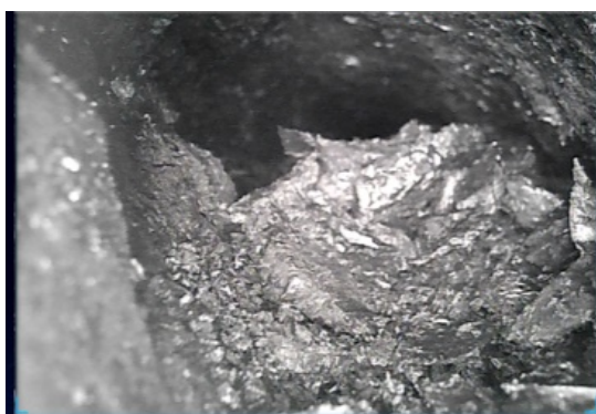
Figure 14. Image of collapsed hole at 39.5 m in 3 # hole.
