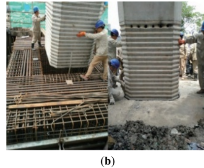
Figure 1. Socket connection: (a) socket connection diagram, and (b) Shanghai Jia Min elevated highway.
