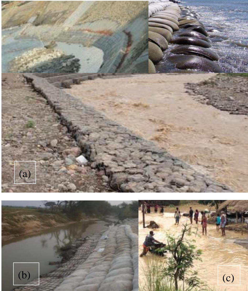
Figure 1. Flood and Anti-erosion works (a) after Singh (2010) [6] , and (b) during lockdown in Bihar April 2020) [7] , and (c) breach in Kamala Balan embankment near Jhanjharpur in July 2019 [8] .
