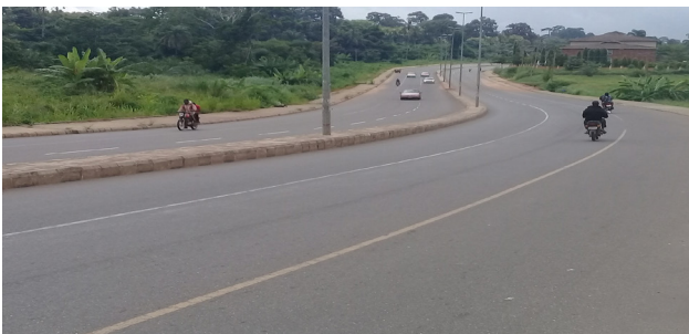
Figure 8. The Akure-Obaile Road Dualisation Project
