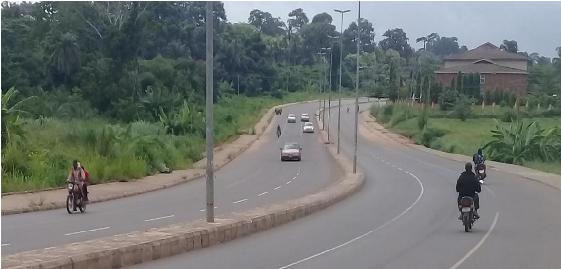
Figure 8: The Akure-Obaile Road Dualisation Project Source: Field Survey (2019)
