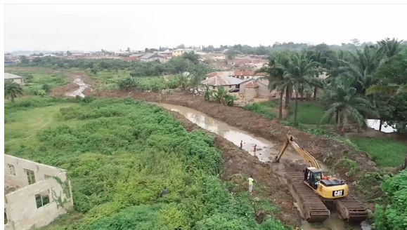
Figure 7. Dredging of Drainages at Alagbaka Ext. II
