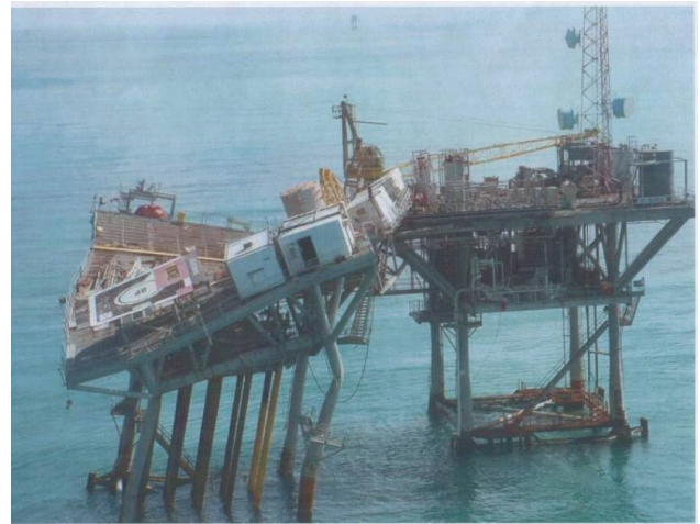
Figure 7.5. Failure at Offshore platforms [15]
