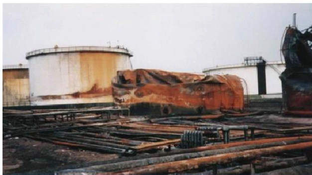
Figure 6.1. The Destroying effect of chemicals in tanks
