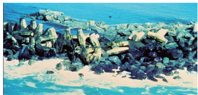
Figure 6.2. (c) Tetrapod type breakwater
