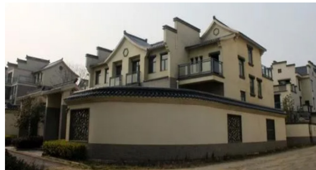
Figure 2. Confusing architectural style in Wan Town.
