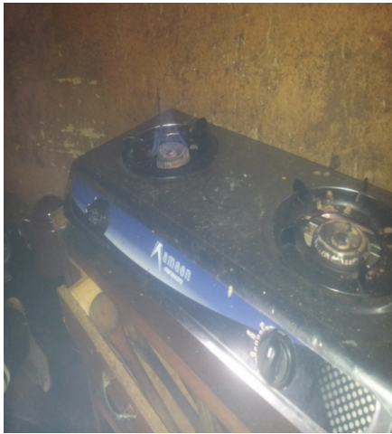
Figure 3a. Self purchased biogas cooking stove
