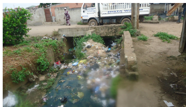
Figure 13. Drainage blocked by wastes in the study area
