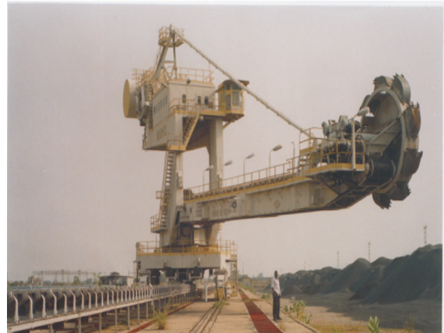
Figure 8. Reclaimer Machine with Iron Ore Concentrate Stockpile
