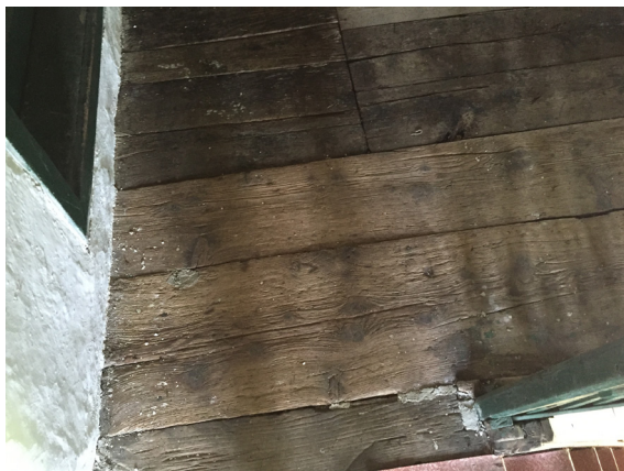
Figure 23. Massive wooden floors in the divanhana
