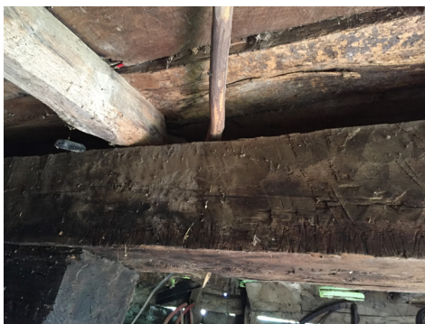
Figure 20. Massive columns and beams of the ground-floor structure are made of chestnut wood
